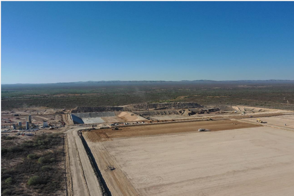
Figure 3: Pond (Pregnant) Liner Installation
