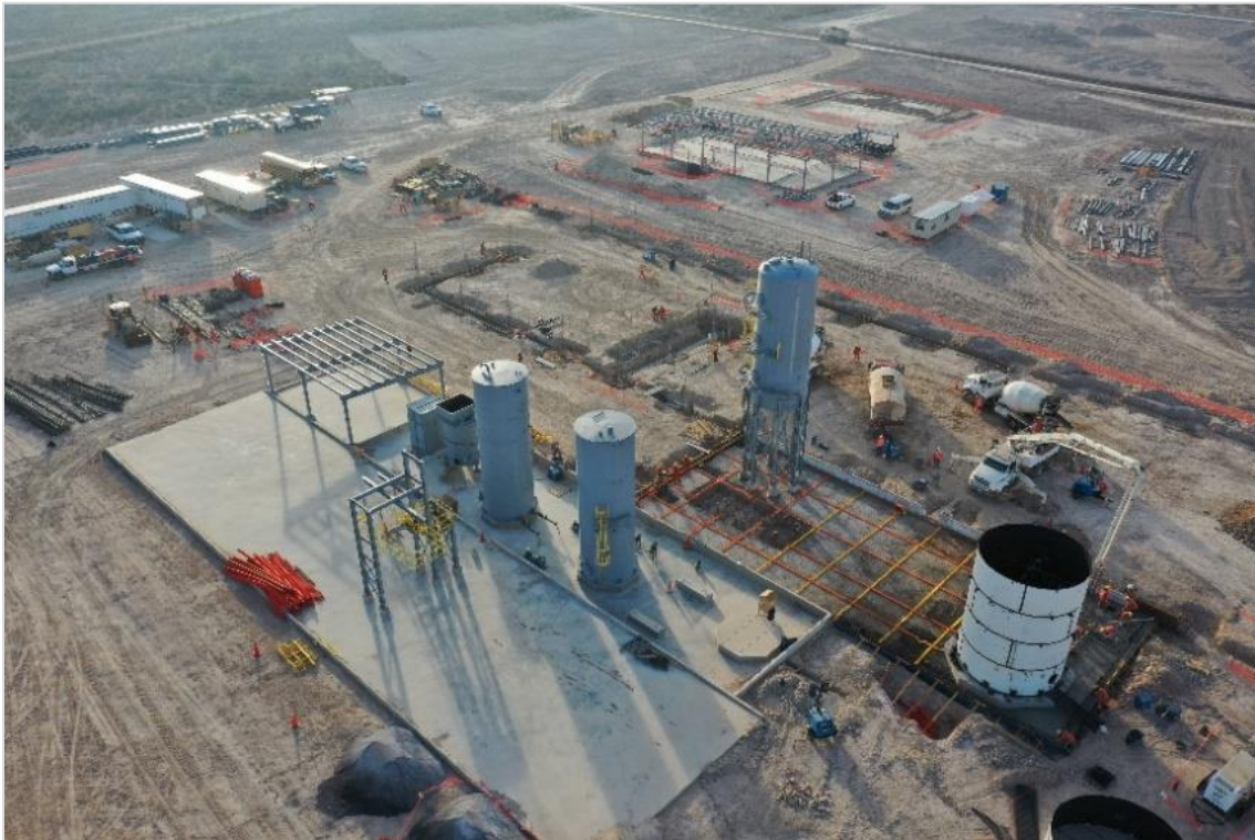
Figure 4: Merrill-Crowe Plant Construction
